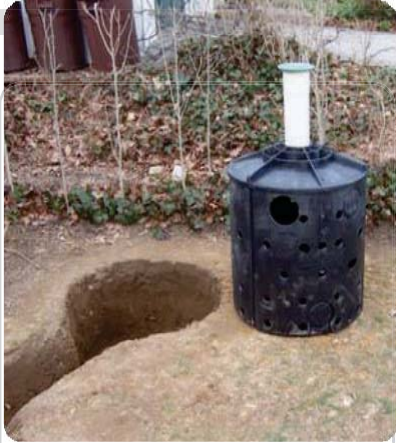
Prefabricated Dry Well Photo Credit: Canale Landscaping
