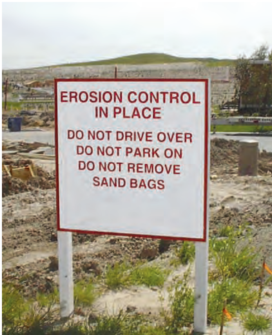
Figure 4. Use signage to help educate construction staff.
