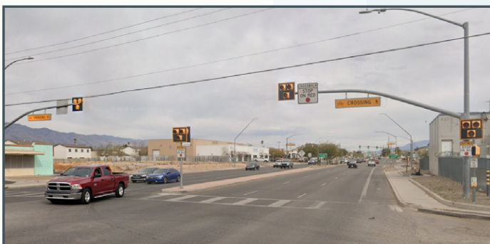
Pedestrian Hybrid Beacon in Tucson, Arizona
